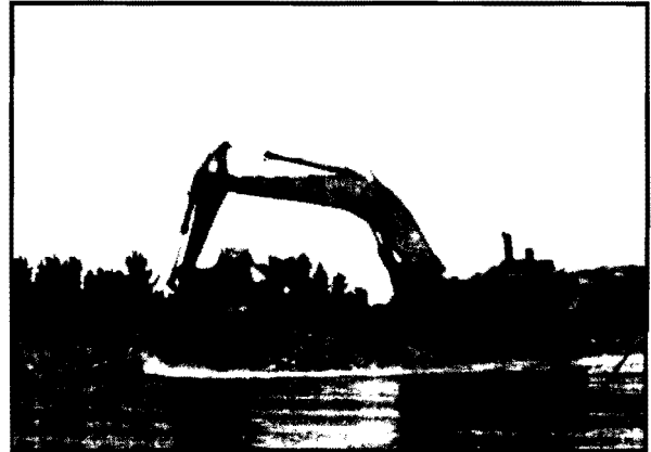
Fig. 22: Mechanical dredging usually raises the dredged material to where it can be seen.
