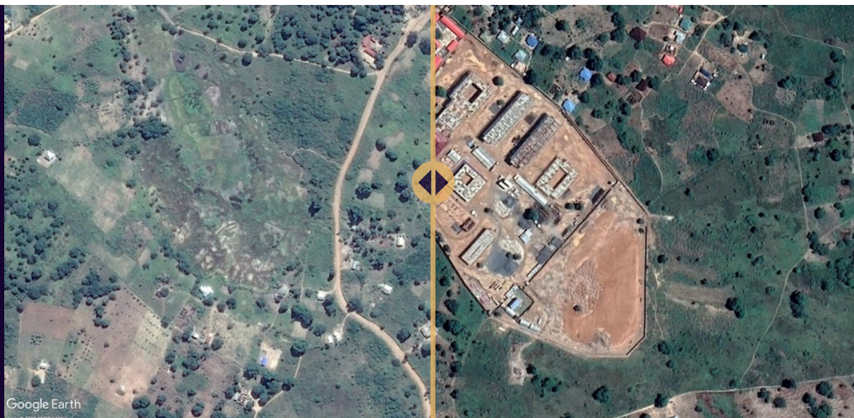
Satellite imagery of the school in 2015 and during construction in 2019 from Google Earth.
