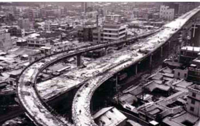
Highway under construction (Seoul Metropolitan Government)
